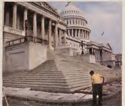
Repairs to sidewalk on the east front of Capitol.
